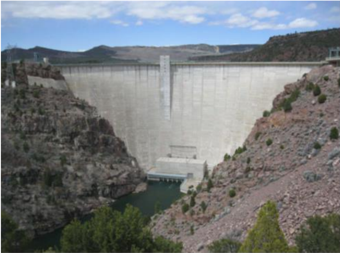
Figure 1-1: USBR's Flaming Gorge Dam and Powerplant
