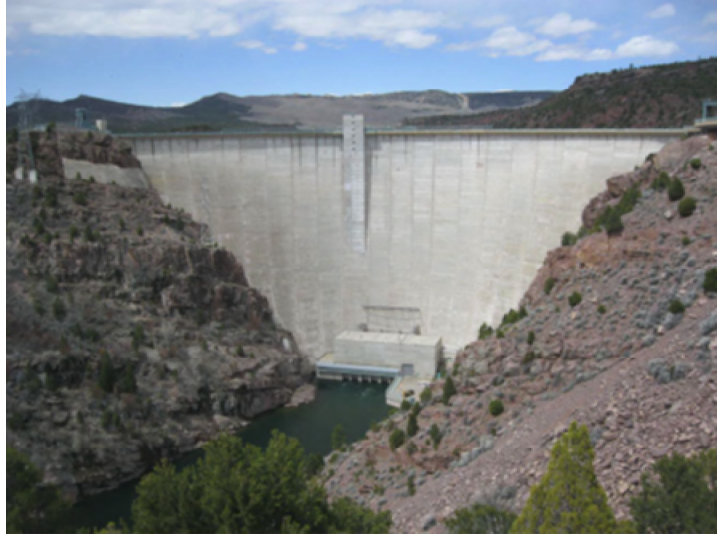
Figure 2-1: USBR's Flaming Gorge Dam and Powerplant
